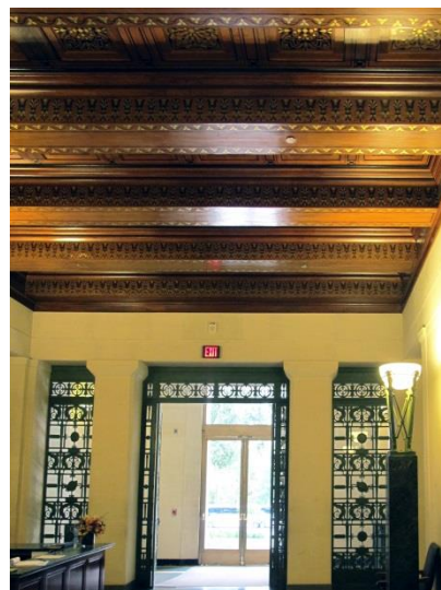
The South entrance interior showing the ceiling woodwork after restoration.
