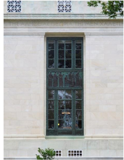
The original South elevation windows after treatment.
