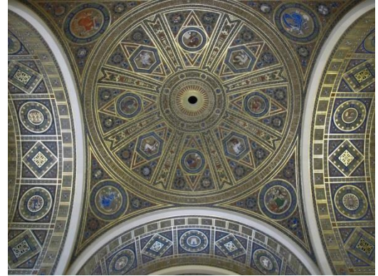
The decorative ceiling in the Great Hall after treatment.
